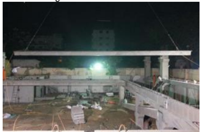
Single Tee Slab Under Erection
