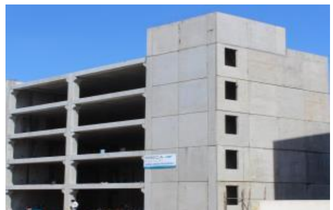
Walls Panels after erection
