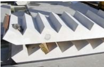
Precast Staircase cast
