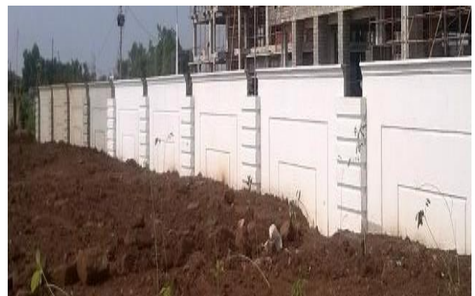
Walls Panels after erection
