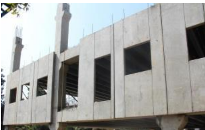
Walls Panels under erection
