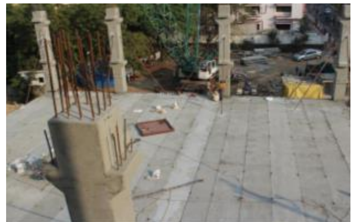
Single Tee Slab Under Erection
