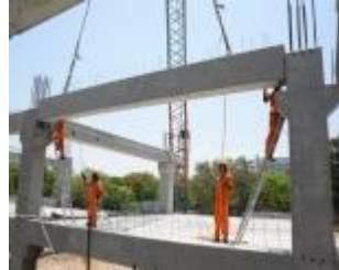
Beam Erection
