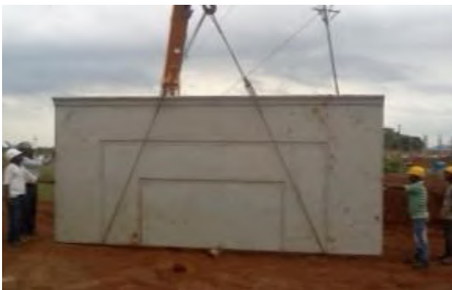
Walls Panels under erection
