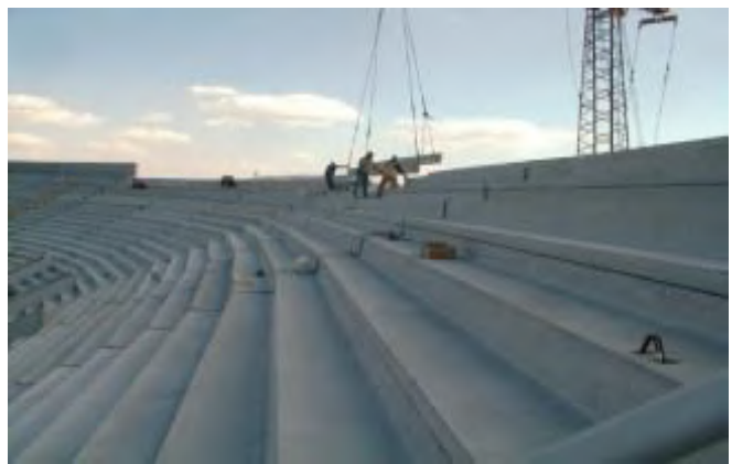
Stadium Seating Sections After Erection
