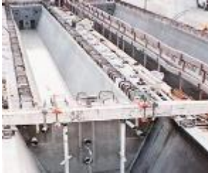
Beam Casting
