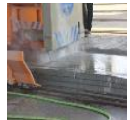
HCS being cut
