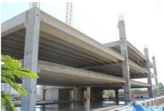
Single Tee Slab – Logistics
