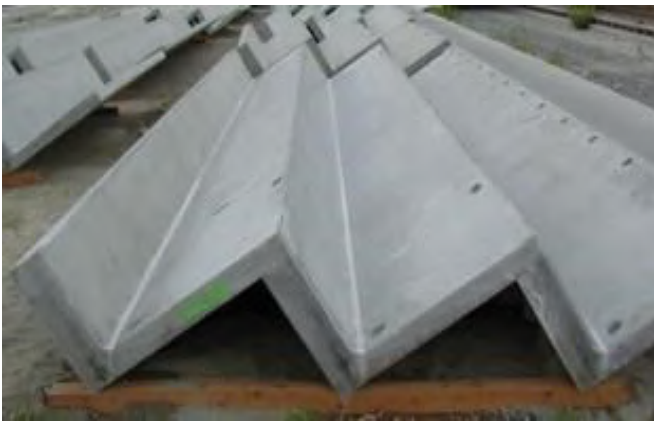
Stadium Seating Sections Before Erection
